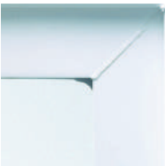
Vinyl sash corner seam
